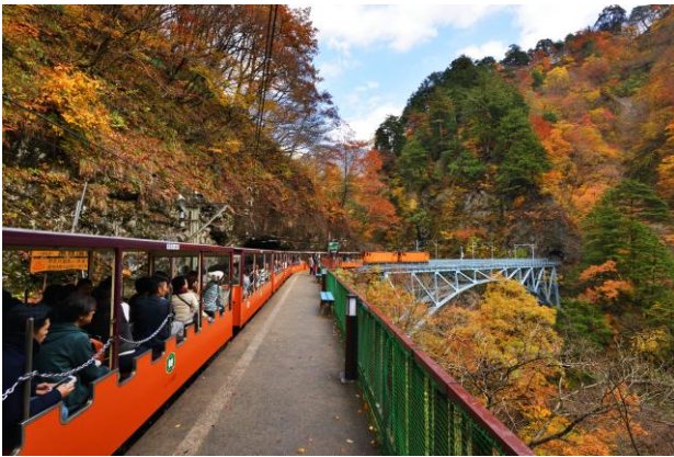
[Kuronagi] At 60 m, Atobiki Bridge is the highest bridge in the gorge.
