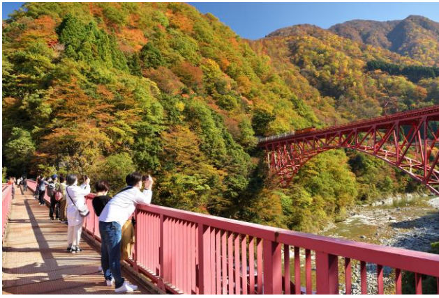
[Yamabiko Bridge] A perfect spot to photograph a trolley train crossing Shin-Yamabiko Bridge.
