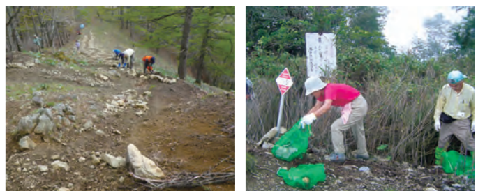
Repairing a Trail
